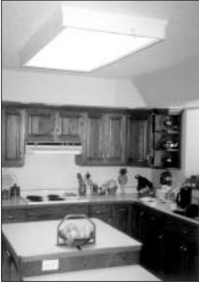
The ceiling light in the kitchen is a four-lamp T-12 fluorescent fixture that was retrofitted with two T-8 lamps, an electronic ballast, and a silver reflector. Light levels are excellent, with 80 foot-candles available below the fixture. The cabinets are birch plywood and solid oak, to minimize off-gassing from wood products containing formaldehyde.
